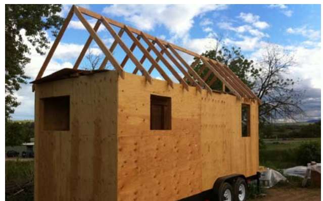
Frame and rough walls on trailer
