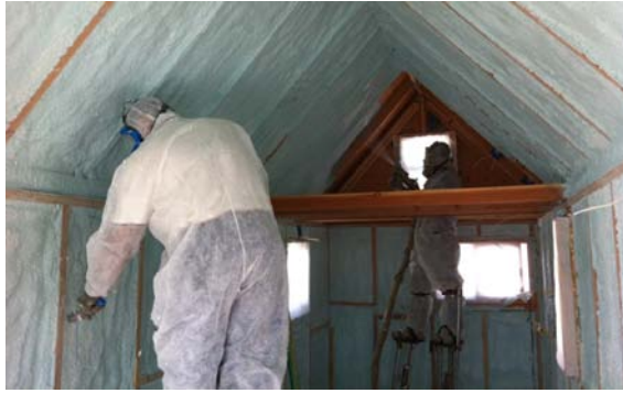
Insulating with blown soy material
