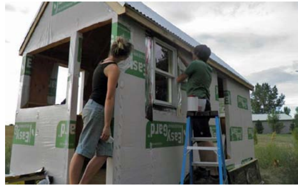
Sheathing on exterior of tiny house
