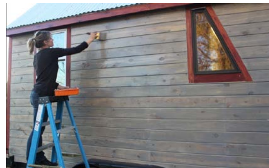
Staining the siding
